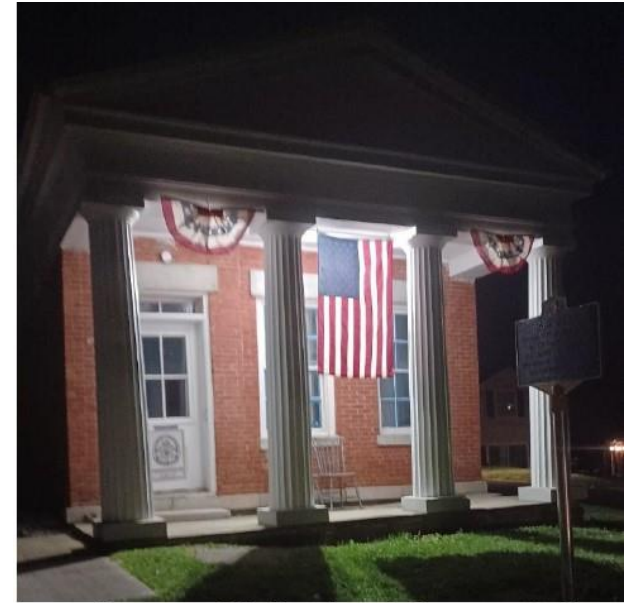
New bunting and dusk-to-dawn lighting installed by Brother Harold Bush, PCC at the G.A.R. Hall in Ovid
